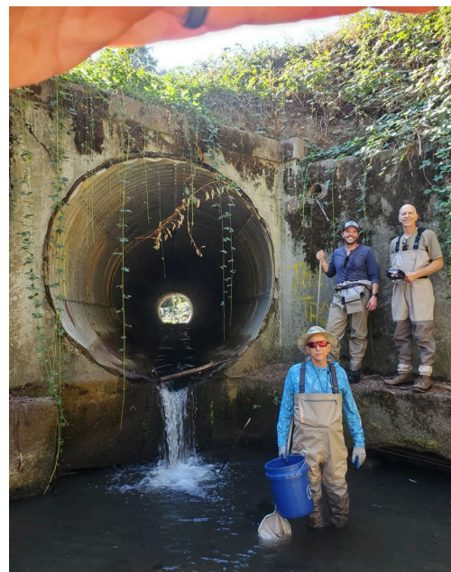
Fruitdale Creek Culvert at Highway 99
