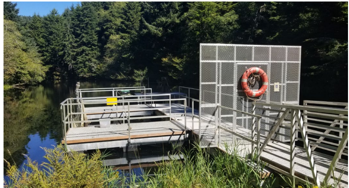
Coho rearing pen at North Depoe Bay Reservoir.
