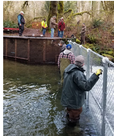
Installing a hanging weir
